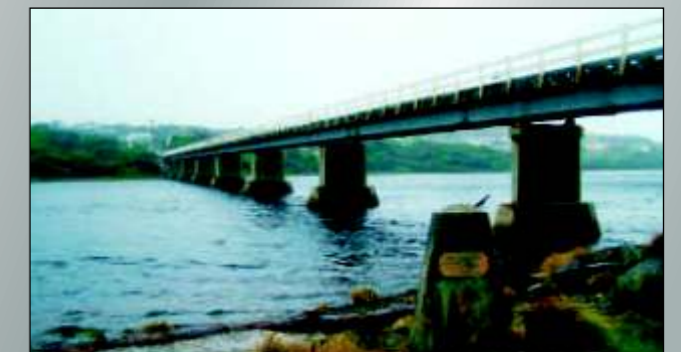
Arthur River Bridge - Australia
