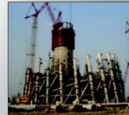
Guangzhou TV Tower - China
